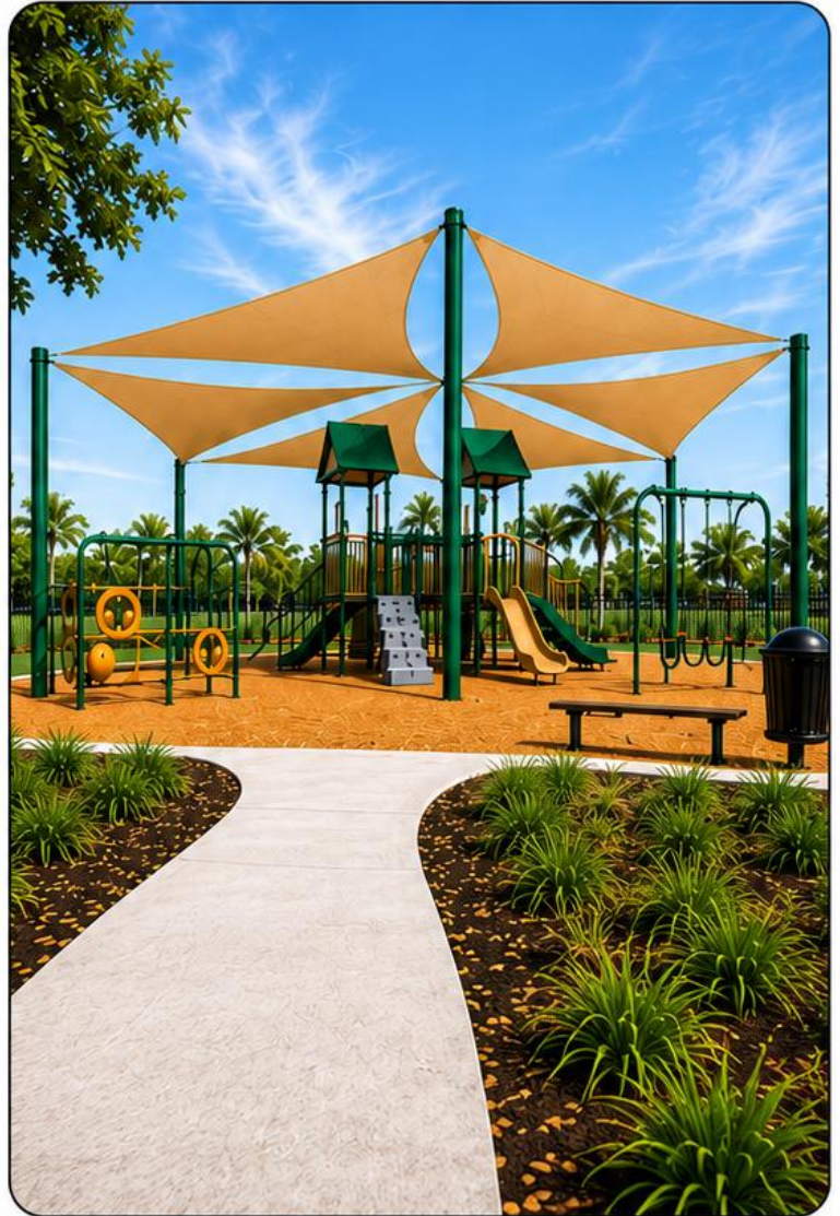
Figure 1. Concept rendering illustrating the proposed six-sail shade structure with seven (7) support posts at the Oakmont Playground.
