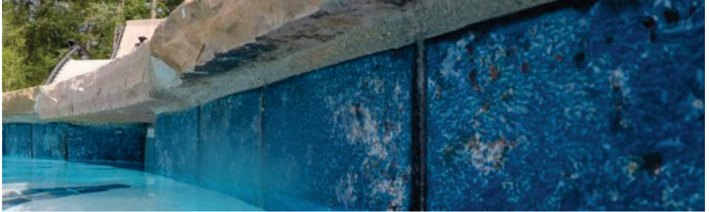
Example showing coping at the top edge of a pool, directly above the waterline tile.
